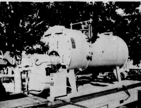
NEW HEATER FOR THE COURTHOUSE - - Workmen were busy this week installing a new heating system for the courthouse, including this Scotch Marine boiler, a gas - fired 80 horsepower unit. Contractor is APCO Boiler Works.
