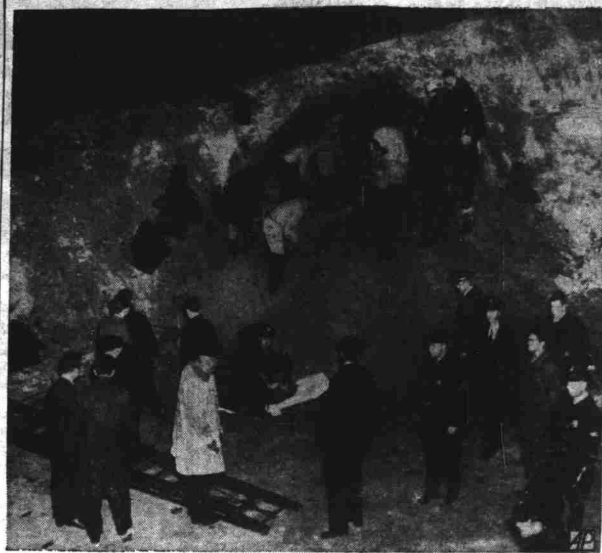
TRAGEDY SCENE—Firemen (top) dig for the body of Francis O'Donnell, 10, as another fireman (foreground) administers to John Whalen, 12, on a stretcher. The two Washington, D. C., boys were buried alive when a tunnel they were digging at play collapsed. Vain efforts were made to revive both boys at the scene and at a hospital. (AP Wirephoto).
