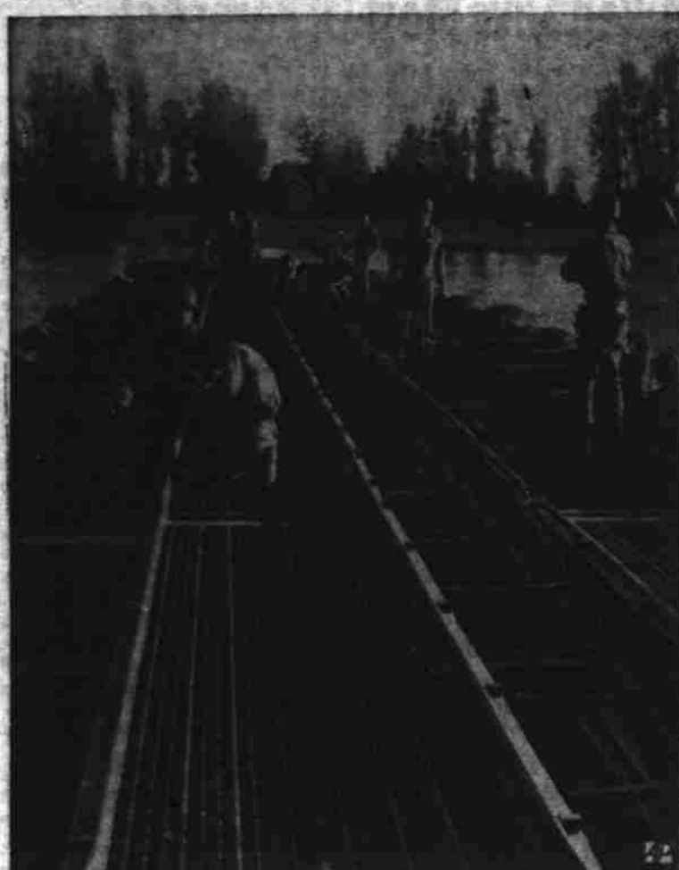
CROSSING THE RHINE — Members of U.S. 1st Engineer Combat Battalion, stationed at Darmstadt, Germany, work on Rhine pontoon bridge between Rheinhausen and Speyer. 6 Men assembled 780-foot bridge in 6 hours and 15 minutes.
