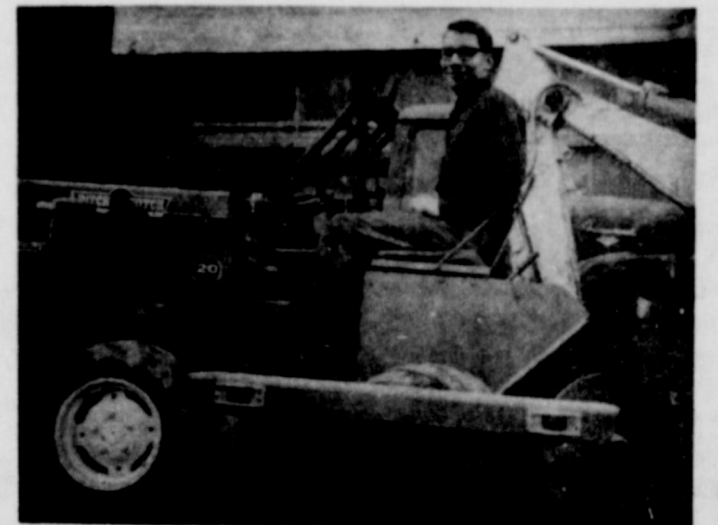
Jerry Maston with ditcher
