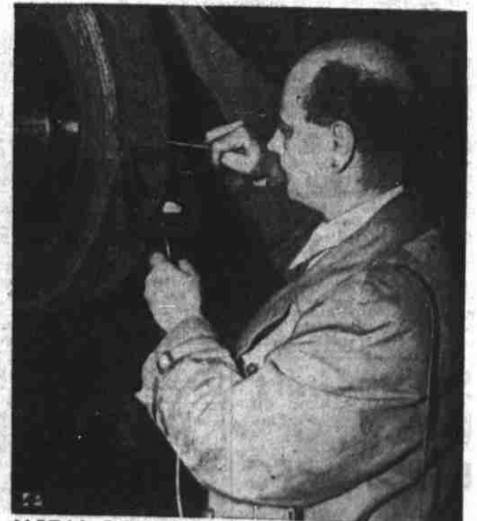
METAL DETECTOR —Electrical instrument developed by Heins Freund of Berlin utilizes a voltmeter which helps to locate hidden nails and other unwanted metal in auto tires.
