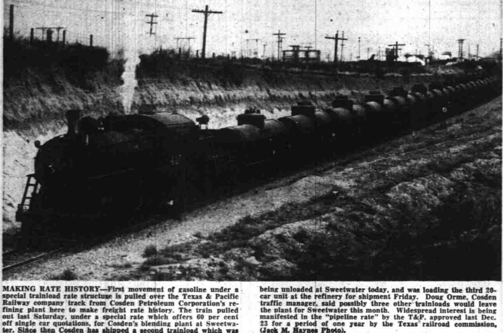
MAKING RATE HISTORY—First movement of gasoline under a special railroad rate structure is pulled over the Texas & Pacific Railway company track from Cosden Petroleum Corporation's refining plant here to make freight rate history. The train pulled out last Saturday, under a special rate which offers 60 per cent off single car quotations, for Cosden's blending plant at Sweetwater. Since then Cosden has shipped a second trainload which was being unloaded at Sweetwater today, and was loading the third 20-car unit at the refinery for shipment Friday. Doug Orme, Cosden traffic manager, said possibly three other trainloads would leave the plant for Sweetwater this month. Widespread interest is being manifested in the "pipeline rate" by the T&P, approved last Dec. 23 for a period of one year by the Texas railroad commission, (Jack M. Hayes Photo).
