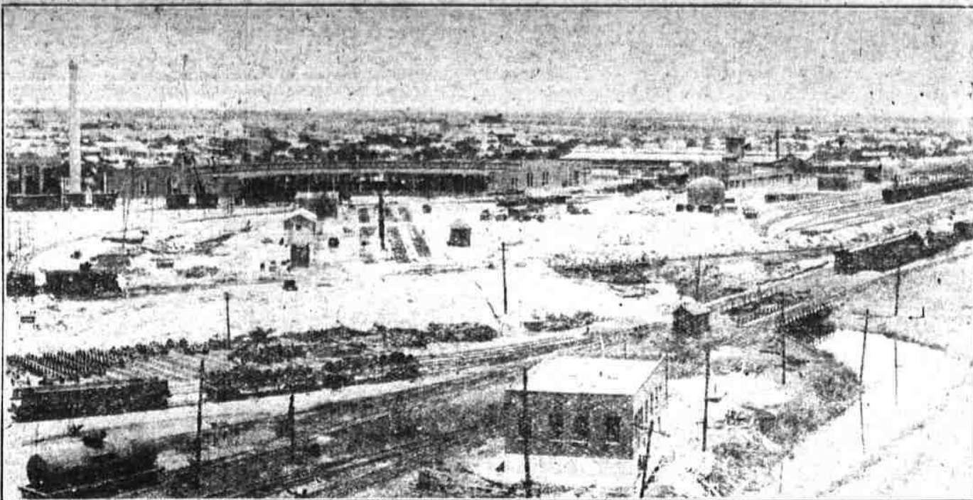
This affords an idea of the completeness of the divisional terminal equipped with latest appliances for servicing locomotives of any type and brass foundry, with a large locker bath building for the house employees. The left of the drop pits used in handling wheels of locomotives. Behind the round house, the 125-foot stack "wing stations." Inspection pit. To the right of the round house are the smith shop and coppersmith's shop and power house. In the foreground is the switchman's shanty. In front of the round house is the three point turntable and nearer the reader are the main power, oil and water "filling stations." Two inspection pits. To the right of the round house are the machine shop, black-
