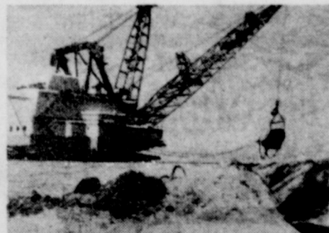
First, the overburden, which is from 40 to 130 feet deep, is removed by this giant dragline.
