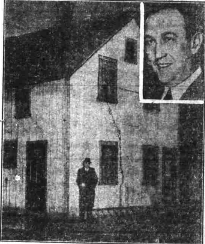
Federal authorities identified the frame house shown above, located in Bensenville, Ill., near Chicago, as the hideout used by kidnapers who held Edward G. Bremer (inset), St. Paul banker, for more than three weeks. The Karpis-Barker gang was sought for the crime. (Associated Press Photo)
