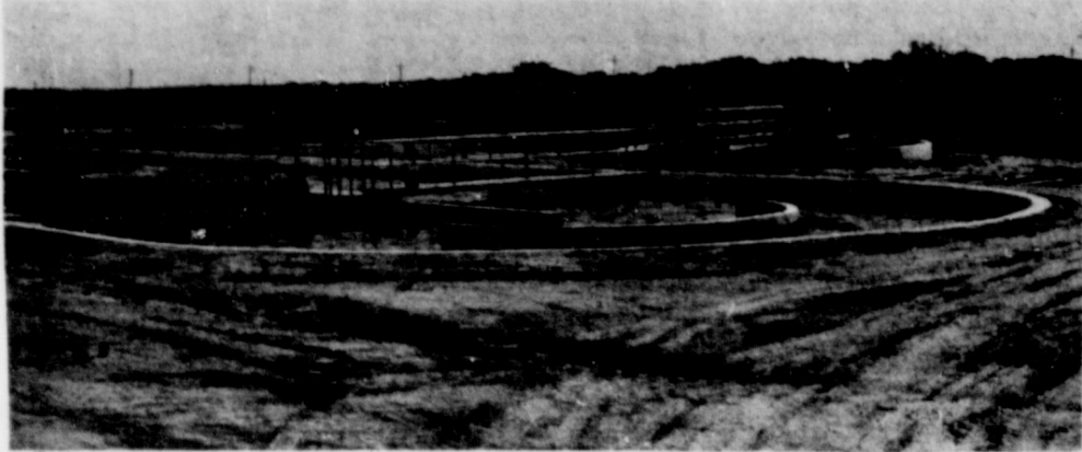
Eastland's new sewage filtration plant is now operating in full swing and according to the above photo, is also running full. (Staff photo)
