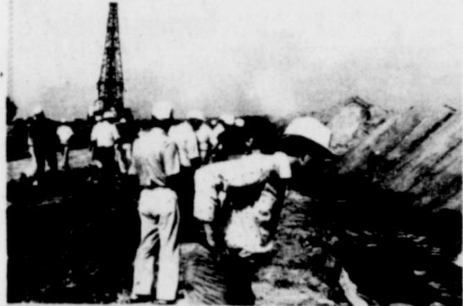
Mike Siebert scans coal ditch
