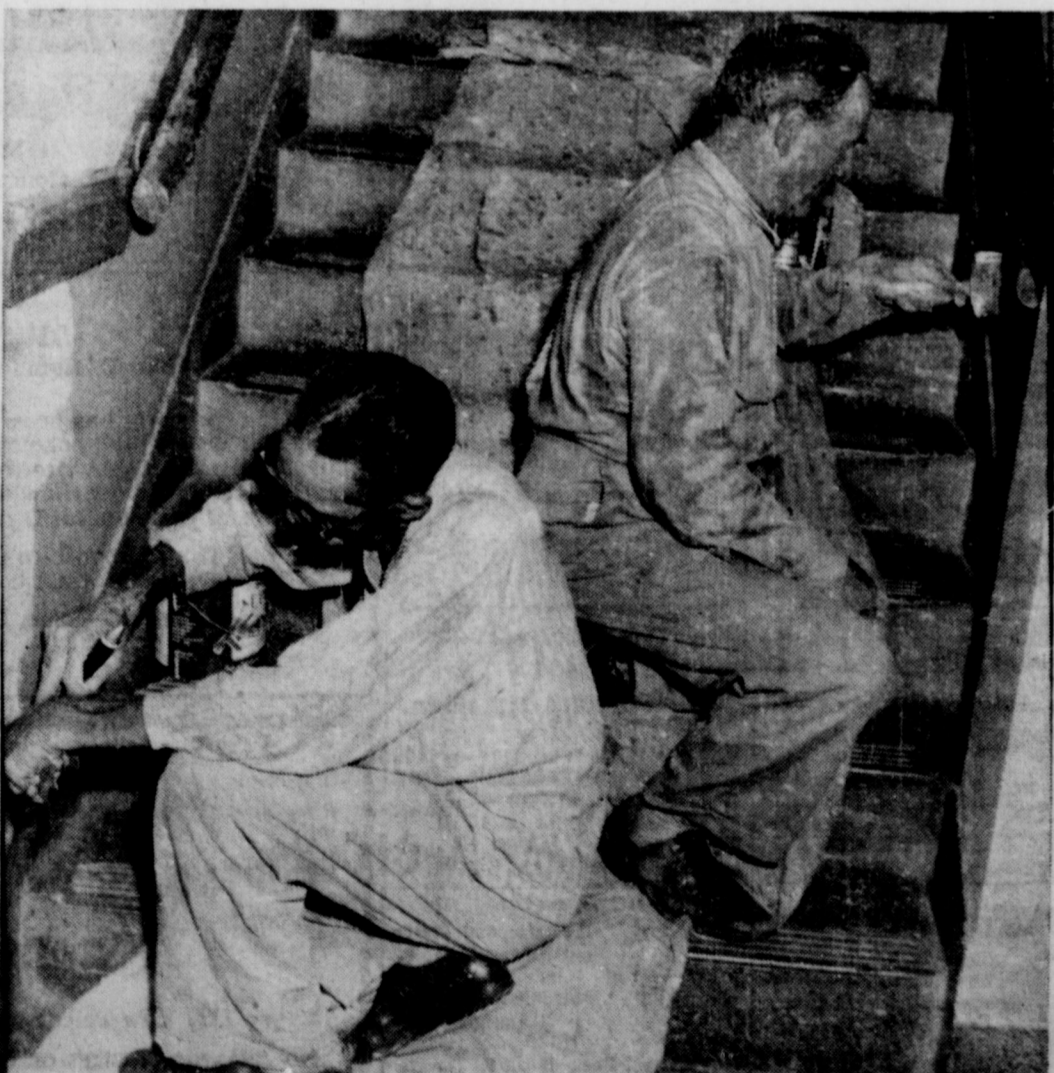
PREPARATION FOR SCHOOL —Seba Williams, high school custodian, and Oliver B. Hogan, South Ward custodian, are shown doing some of the painting which will ready Eastland schools for their August 28 opening. Refinishing desks and floors and doing general repairs have given the men a busy summer. They have been assisted by Marlon Asher and George Prestridge. Pre-registration for the second through the eighth grades will be Aug. 25 from 9 a.m. to 12 a.m.
