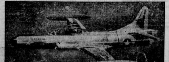
"STARFIRE" INSPIRES SWISS-USAF's F-94C Starfire, above, has apparently inspired deof Switzerland's first home-built jet pursuit plane. Swiss P-16 has similar air intakes, same type wing and similar backbone ridge from pilot's canopy to tail assembly.
