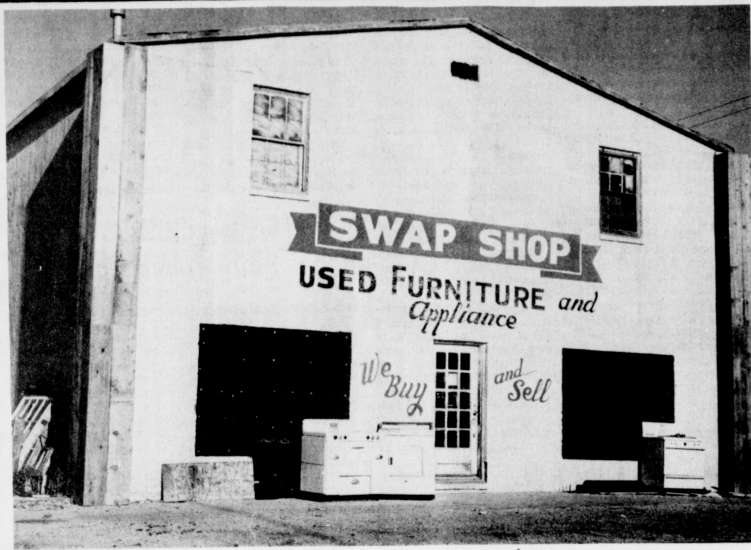
RENOVATION PROCESS BEGINNING--This former site of the Swap Shop is being completely renovated and will feature Mexican architecture and decor when the doors are opened in the next few weeks. Gary Miller has purchased the location and is spending in excess of $70,000 in the renovation process before he opens the doors to Muleshoe's newest steak house. He said fine steaks will be a feature of the new business.
