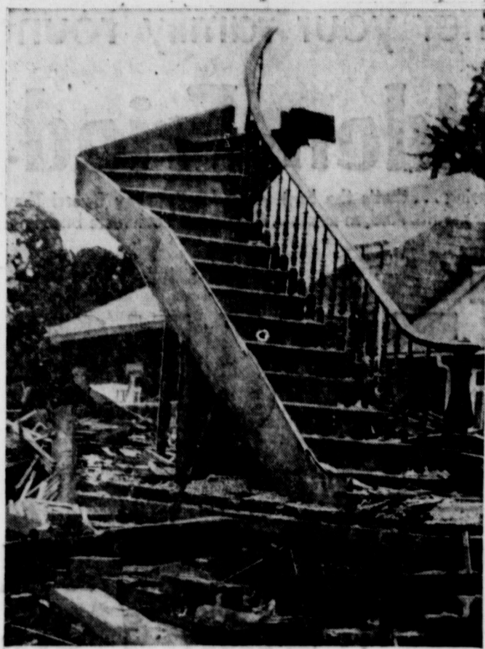
FLIGHT CANCELED —This stairway would lead any climber to an unhappy landing in Crawfordville, Ind. It was the last portion standing of a home under demolition.
