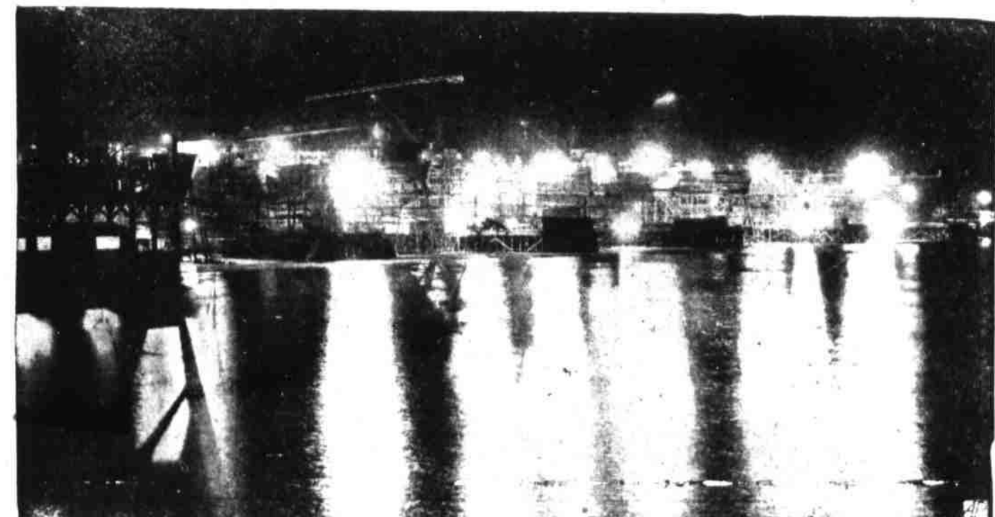
NIGHT SHIFT TAKES OVER —Welders' arcs and floodlights give a holiday atmosphere to this night scene along the West Ways at the New England Shipbuilding Corporation yards located in South Portland, Maine.
