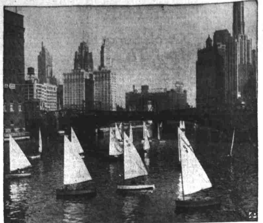
RIGHT THROUGH CHICAGO — Dinghies pass under Dearborn Street bridge on Chicago River during Columbia Yacht Club's Frostbite Regatta, last of the sailing season.
