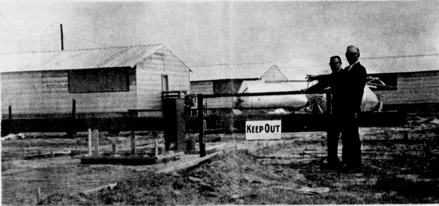
MILL SITE--Don Harmon, left, and Harmon Elliott point out the site of a feed mill at Muleshoe Swine Breeders Inc. The mill will be erected within the next week and ten days and will join some of the buildings already completed in the background at
