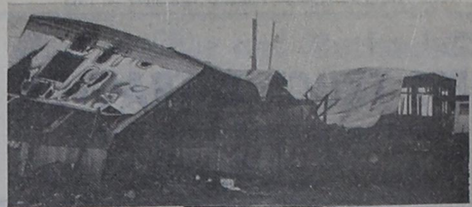
HOME DESTROYED: The trailer home of Mr. and Mrs. Ronnie Alley was destroyed early Wednesday morning. The Wheeler Volunteer Fire Department was called at 2:56 A.M. but were unable to save anything. The cause of the fire is unknown.
