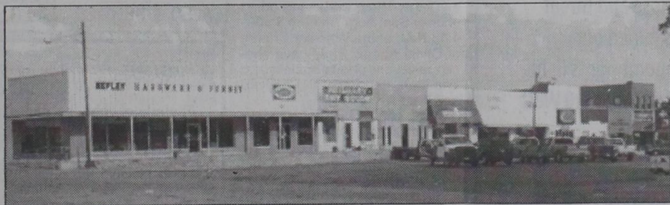
West Side of 400 South Main, 2005
