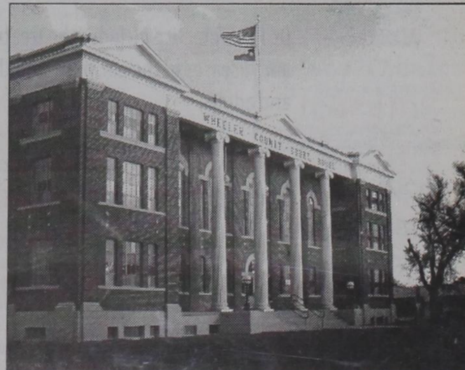
Wheeler County Courthouse 2005 After Renovation
