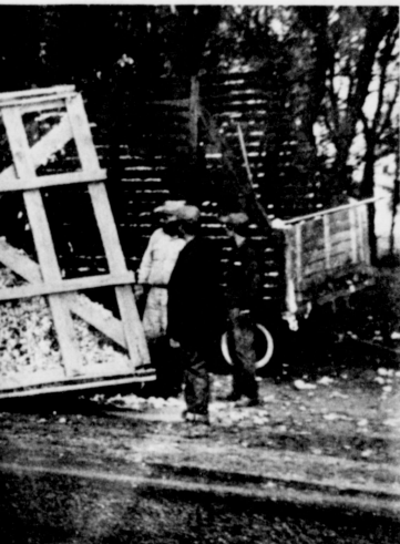
HARVEST-TIME HAZARDS--Pat Childers was hauling a load of cotton to town Wednesday afternoon when a right wheel bearing went out locking the right wheel and dumping this trailer load of cotton along the highway about two miles northwest of Muleshoe on Highway 214. Employees from the Childers farm are shown pondering how to go about setting the trailer upright again. Incidentally, it was Childers' last load of cotton for the year which was dumped. It got all wet as it rained in the Muleshoe area Wednesday night, and a light rain was falling at the time the picture was made Thursday morning.
