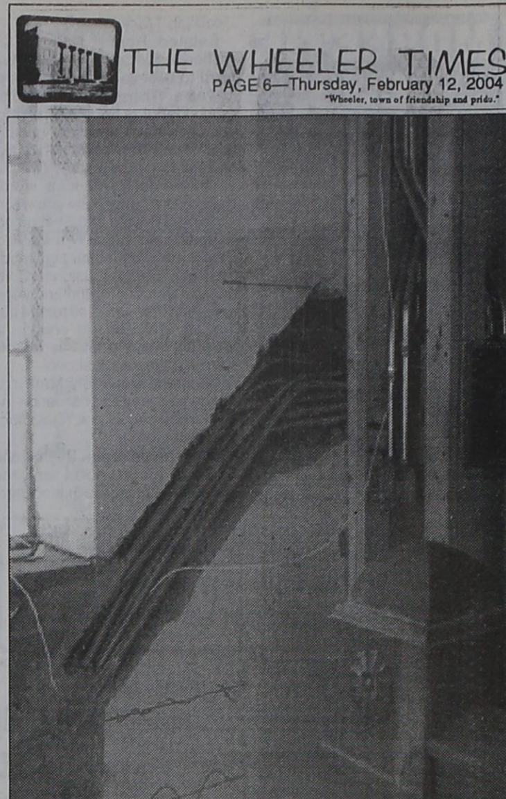
WIRING: The work on the Wheeler County Courthouse continues at a rapid pace. This picture shows how the wiring for the telephone lines, electrical lines, etc. are run in the walls and ceiling. The walls and most of the ceilings have lines like this running in them. The lines will be bricked and plastered over.
