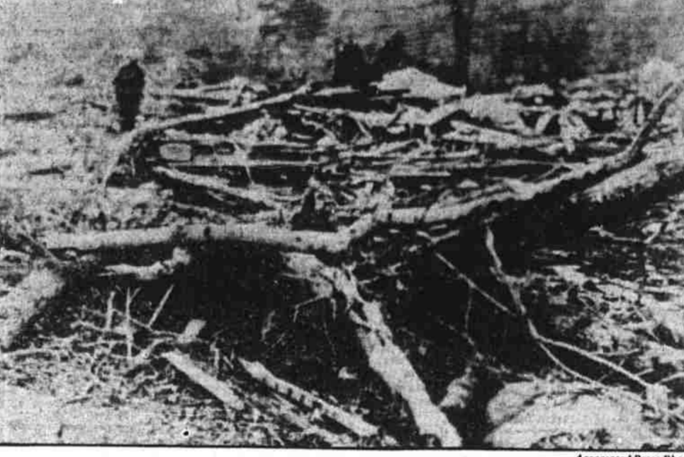
This Associated Press telephoto shows the wreckage of a house in Cartersville, Ga., in which seven persons narrowly escaped death. This was typical of destruction caused by tornadoes in several southern states.
