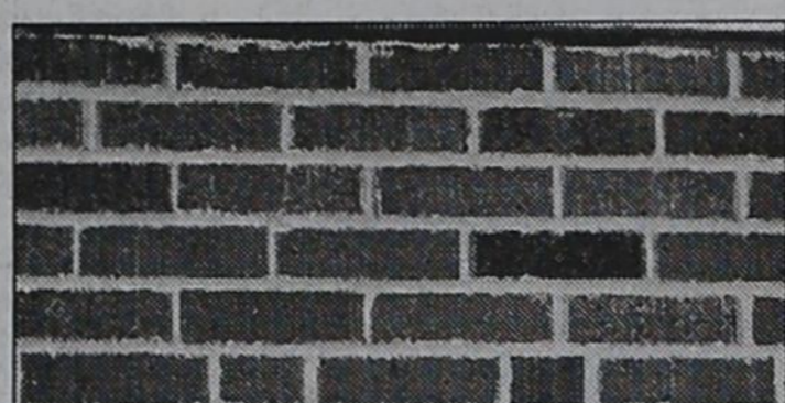
After the mortar has been replaced. —Photo by Rob Schaffer
