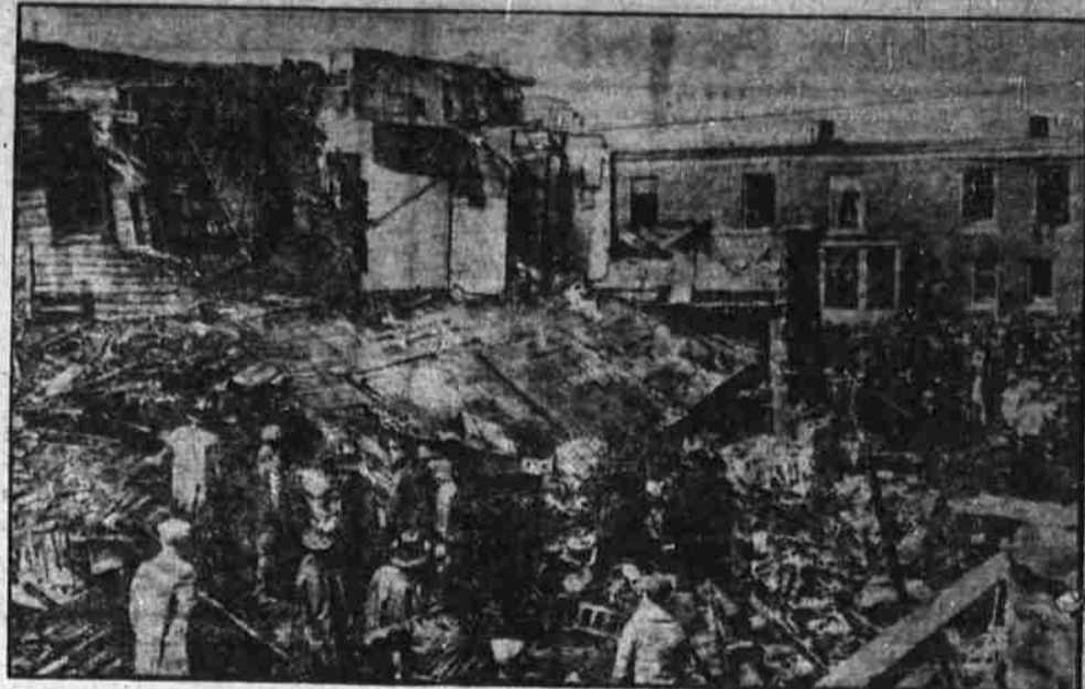
Associated Press Photo One person was killed and 24 others injured, several seriously, when a gas explosion in a Detroit plumbing shop wrecked four store buildings and a flat in suburban Highland Park. The shop where the explosion occurred is shown here. A broken gas main was blamed.
