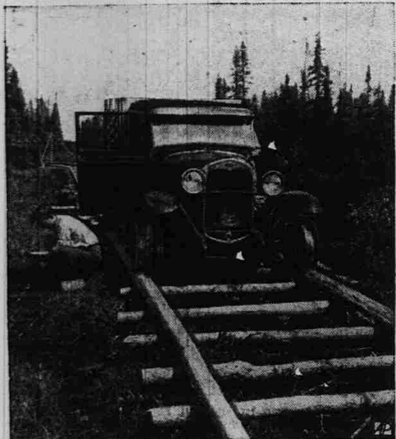
WATER FOR ENGINE —The "engine" on the Bourlemarque Central railroad, built of saplings to reach seven miles across deep swamps in a new gold strike region of western Quebec, pauses to dip swamp water for his engine.
