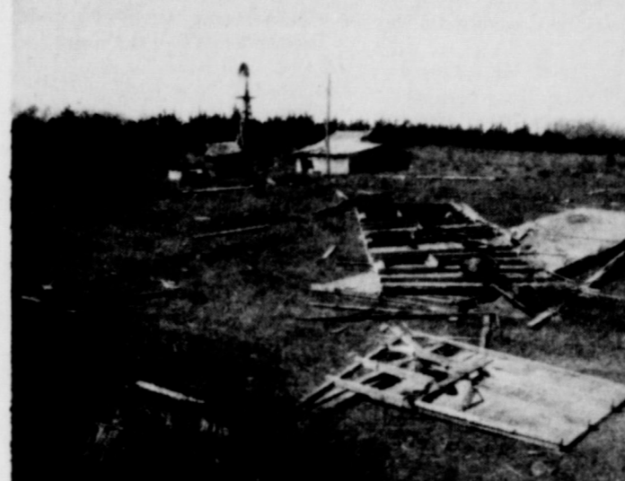
WIND OR TWISTER: A cloud which passed over the Wheeler area Monday afternoon brought with it a strong wind or small twister which damaged property 4 miles south of Wheeler and 3 miles southeast of Wheeler. A shed (pictured above), belonging to C. E. "Shorty" Later, was ripped from its foundation and scattered over the surrounding area. As the cloud moved north east it uprooted some trees at the home of Mr. and Mrs. Cleo Gaines. The damage occurred around 4:00 P.M.
