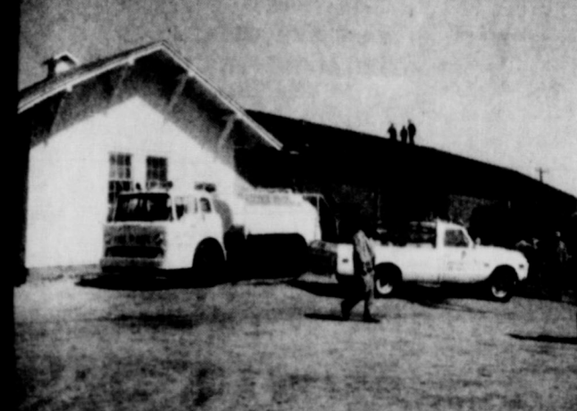
TUESDAY AFTERNOON FIRE: Fire units from Wheeler, Briscoe, Allison, Mobeettie and Canadian were called to Briscoe School Tuesday afternoon to fight a fire in the gymnasium. The fire was extinguished and the structure suffered by smoke and water damage.
