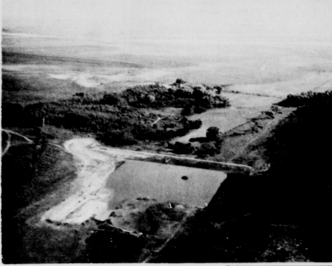
Ponds such as this one constructed by J.T. Johnson, provided stock water, assist with flood control and have potential for good recreational facilities.
