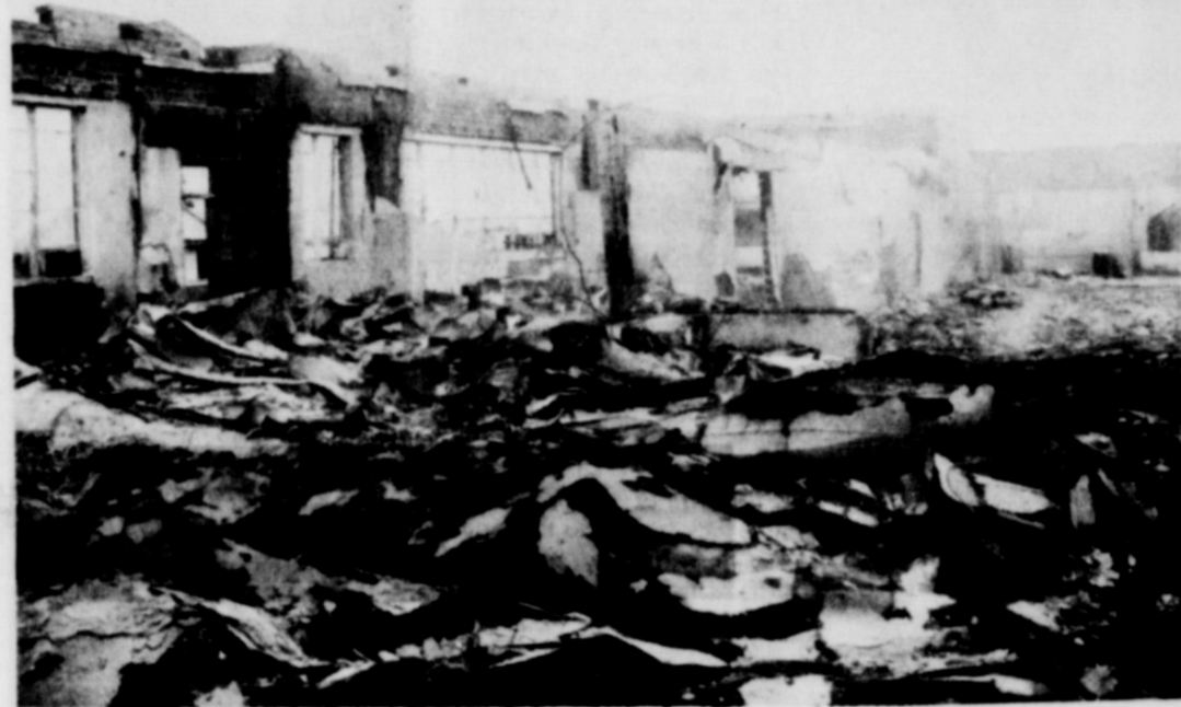
INTERIOR: Friday, 78 students and their instructors studied and played inside these walls, looking forward to the end of another school year only two weeks and three days away. Fate stepped in and left the students and teachers without classrooms and materials. The exterior walls and one interior wall was all that remained of the tile and brick structure after a fire early Monday morning.
