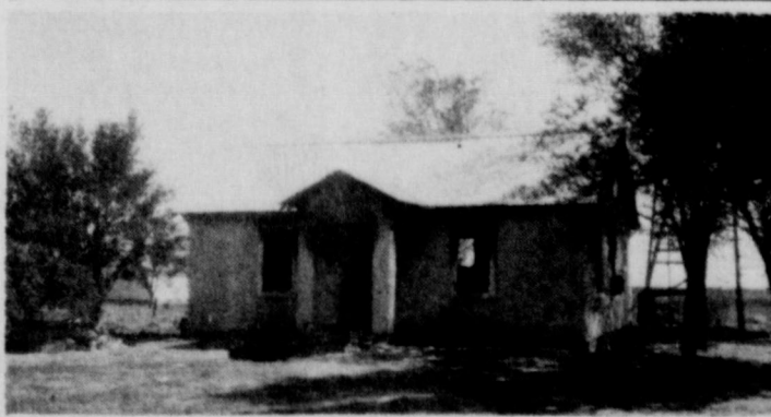
HOME DESTROYED: The home and contents of Rev. and Mrs. Bob Ming was destroyed by fire at Briscoe about 12 midnight Saturday. The fire was discovered as the couple returned from attending services at Mobeetie. The Briscoe, Allison and Wheeler fire departments fought the blaze. Rev. Ming is the pastor of the Assembly of God Church of Briscoe, and has been in Briscoe about a year. The cause of the fire which destroyed the two-bedroom stucco house was not determined.
