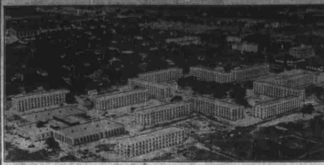
Final touches are being given the twelve new dormitories and dining hall at Texas A&M College and all of the buildings will be completed in time for the opening of school on Sept. 22. The new dormitories will have 1210 rooms and house 3250 of the students expected to attend the college this year. For the first time in several years there will be space enough to care for the entire student body in the halls or in the several project houses on the campus.
