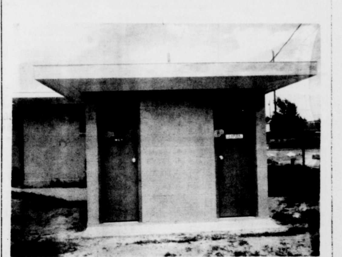
PARK RESTROOMS: Two new restrooms have been added to the city park area. They are located at the swimming pool on the west side. They are for the entire park, baseball field and pool areas use. The City built the two 5'x8' rest rooms. Jake Holcomb was the contractor. Each rest room is fully equipped and has a steel door.
