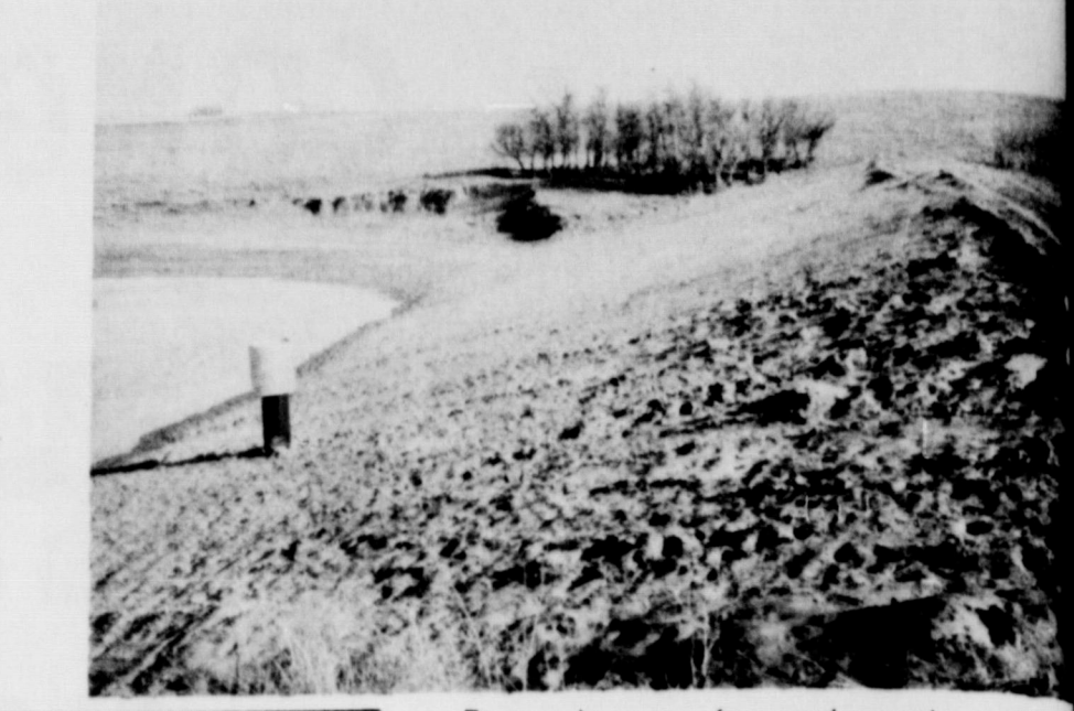
Picture shows new farm pond recently completed on ranch east of Wheeler. This pond was constructed across a live water stream and will have a good supply of stock water at all times. Draw down tube will keep permanent water at constant level, with flood water storage between draw down level and emergency spillway level. This will protect spillway from erosion. Additional stock water is always good to help obtain a more even distribution of grazing. There are many good pond sites in Wheeler county and if you are interested in having one constructed, contact your Soil Conservation Service office in Wheeler.
