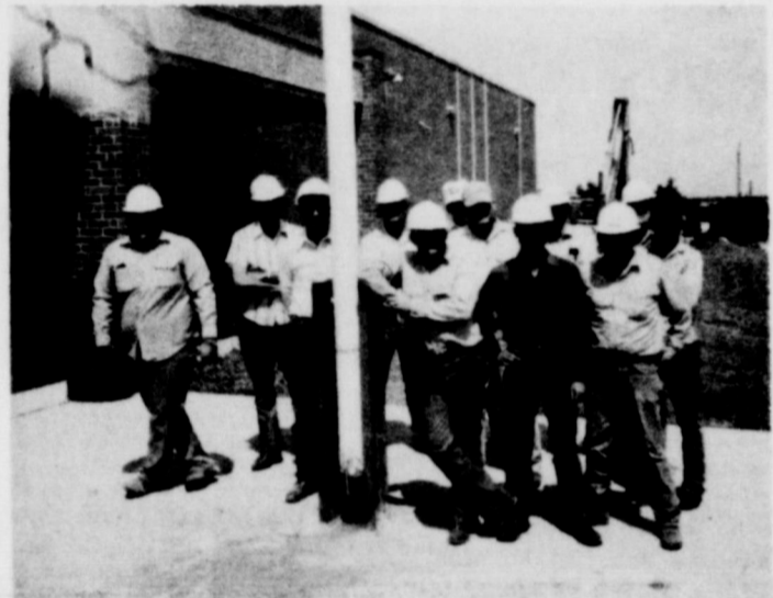
THE LASOR FORCE: Natural Gas Pipeline Employees helping to erect the flag pole are (l to r) Sam Montgomery, M. D. Dutton, pipeline forman, Bob Patterson, platformer, Gene Harrison, Bob Vanpool, Neil Rogers, L. K. Bunch, Bill Ridgeway, Riley Atwood, M. A. Mendoza, John Meadows, and Don Denton.
