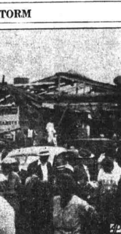
This is a sample of the damage done in Charleston, S. C., by a sudden storm which killed nearly 30 persons. The wreckage shown here is that of the historic old City Market and it is stocked around the Harriott Pickney Home for Seamen, which escaped major damage.
