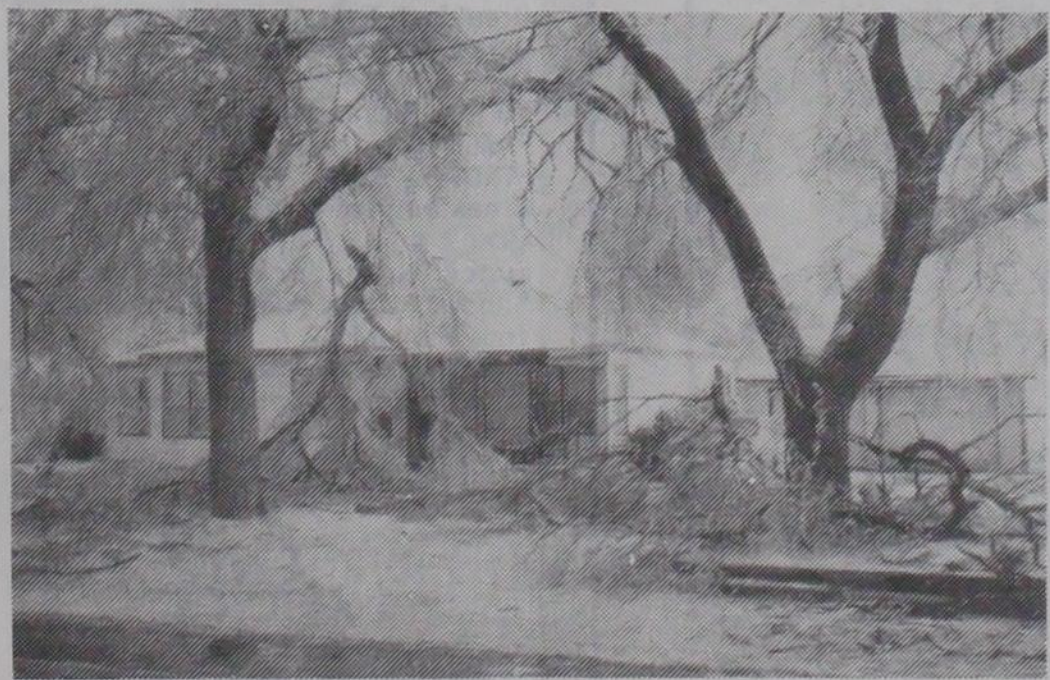
TREE DAMAGE: The Steve Guthrie residence on the south end of Main Street has the drive covered with tree limbs, broken on the ice over the weekend. Wheeler received 1.67 inches of moisture from ice, sleet and snow which fell Saturday evening thru Sunday.
