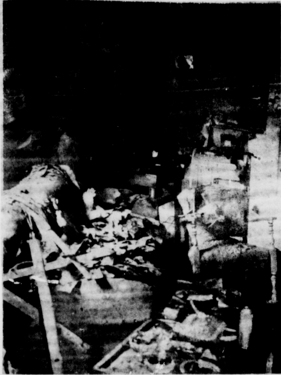
HEAVY DAMAGE: The home of Mr. and Mrs. J.B. Mann received severe fire and smoke damage Sunday evening. The Manns returned home from Church around 9:00 p.m. to find their house ablaze. The furnishings in the livingroom were completely destroyed, and the rest of the house, furnishings and clothing received heat, smoke and water damage. The town is coming to the aid of these elderly residents. A collection was taken up Monday with a total of $250 collected. Anyone wishing to make a contribution can do so at Daughtry's Ben Franklin Store. In
