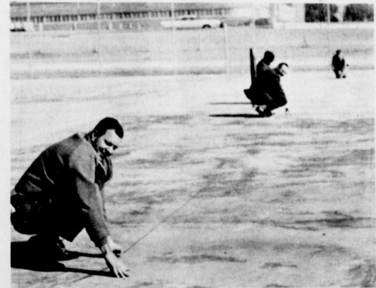
NETS NEXT ---Tom Jinks, high school principal; Superintendent Neal Dillman and school employees Bill Williams and Otis Blylock are pictured measuring and preparing to mark the newly constructed tennis courts south of Muleshoe high school. When the marks are painted on the concrete slab, nets will be put up and the court open for tennis players. All work has been completed with the exception of this phase.
