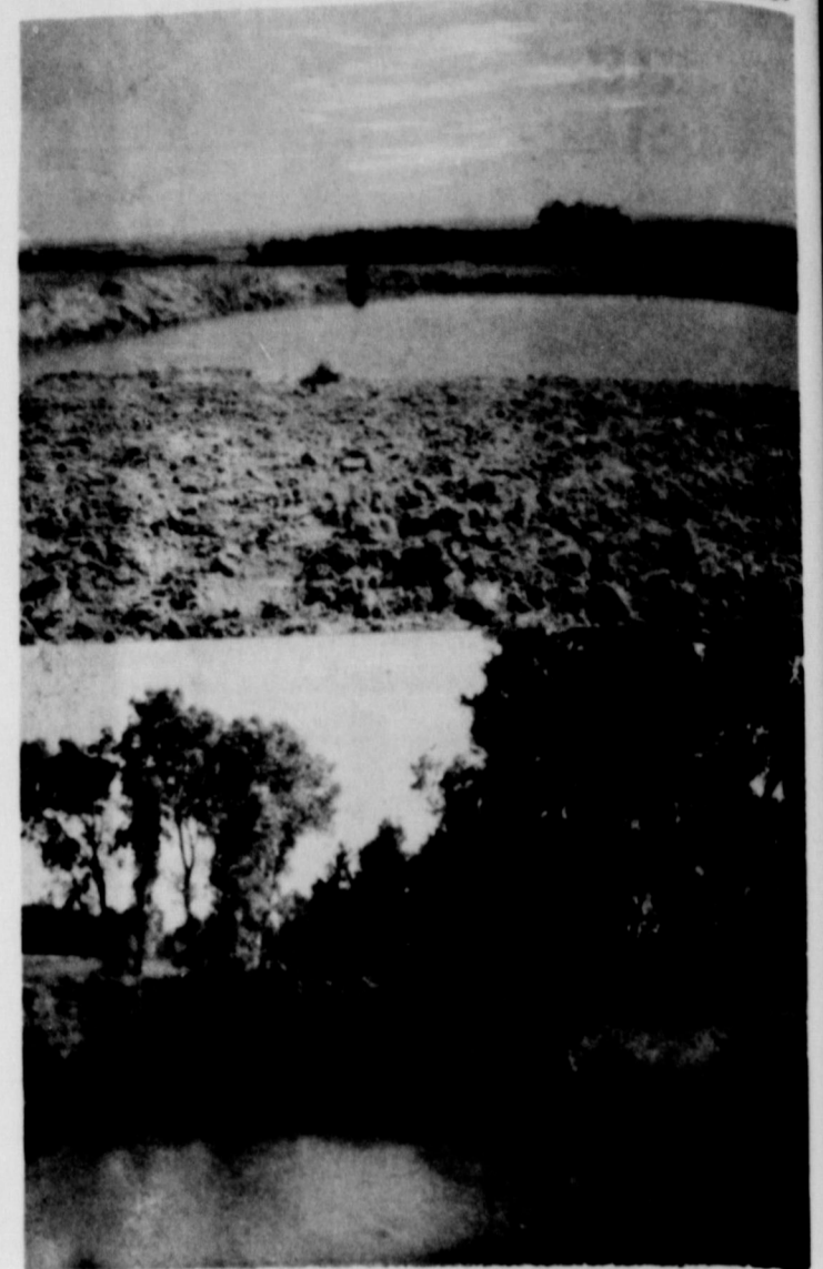
Shown Below: Seep Type Pond constructed on O.E. Chenoweth property. Dimensions: 60X90X9.5. Shown Above: Seep Type Pond constructed on Wiley McCroy property. Dimensions: 60X90X12.
