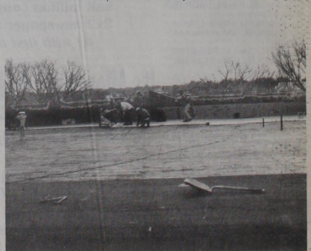
The crew starts to put down the felt paper.
