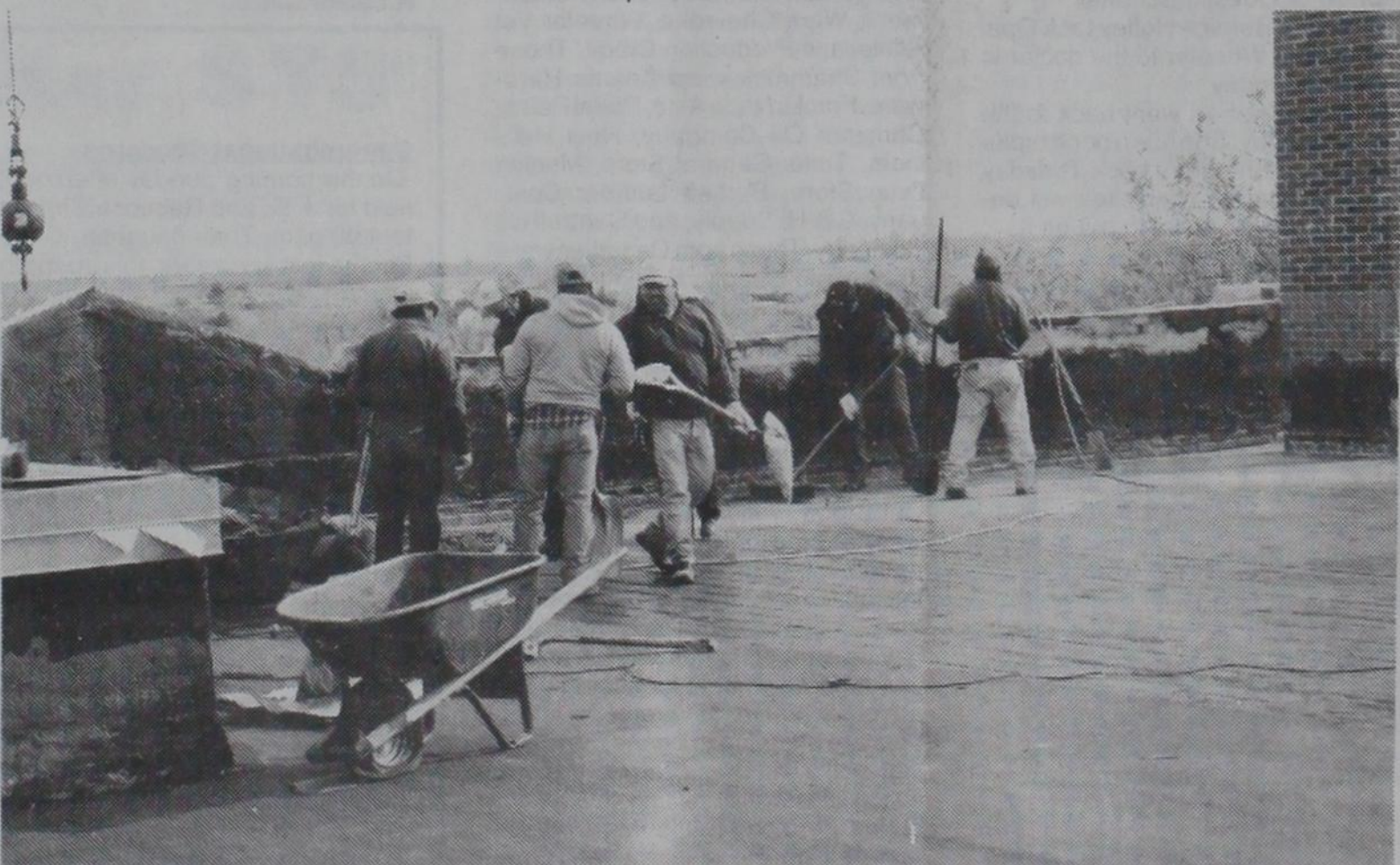
A crew of 19 men worked on the roof at one time.
