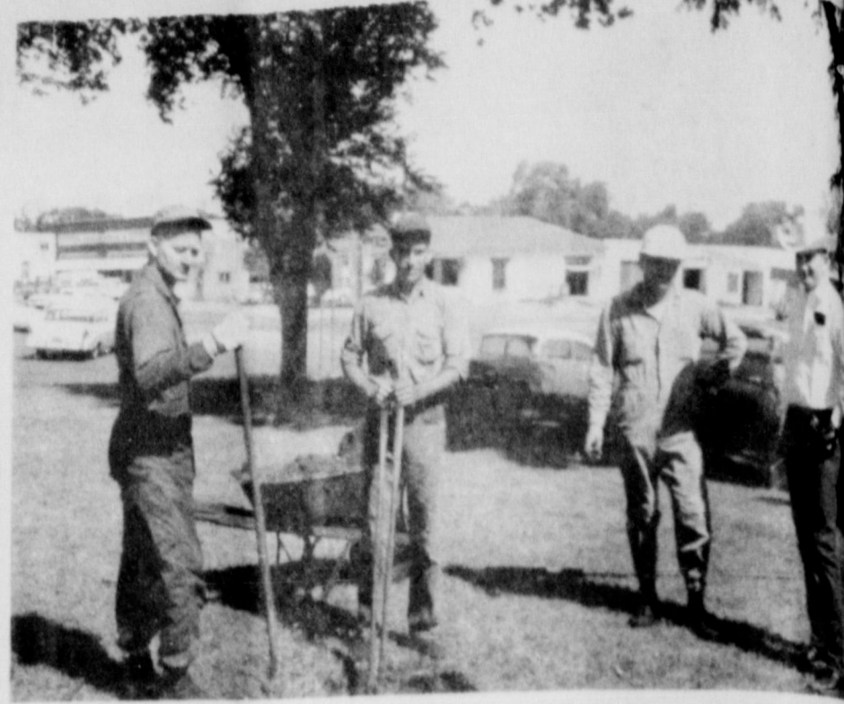
WORK BEGINS: The base for the flag pole on the Court-house Square was set Wednesday afternoon by three men from the United Carbon plant at Shamrock. The pole and base are sponsored by the Wheeler County 4-H Council. The pole is being donated by United Carbon; it is 92 feet high with the diameter ranging from 8" to 4". Wheeler Redi-Mix Concrete donated the concrete to form the base for the pole.
