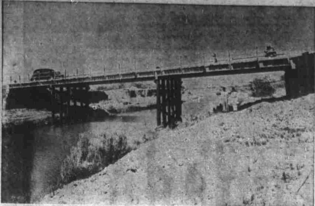
Pictured above is the new bridge across Beal's creek in the southeast portion of Howard county, an important structure because it links the Snyder and Chalk oil field areas, opening a flow of traffic between the fields. A 100-foot, three span structure of steel and wood, it was constructed by the county at an outlay of about $7,000, and was formally accepted by the commissioners court last week. Supervising the job was Commissioner Arch Thompson, pictured below, in whose precinct the bridge is located. (Bridge photo by Kelsey).
