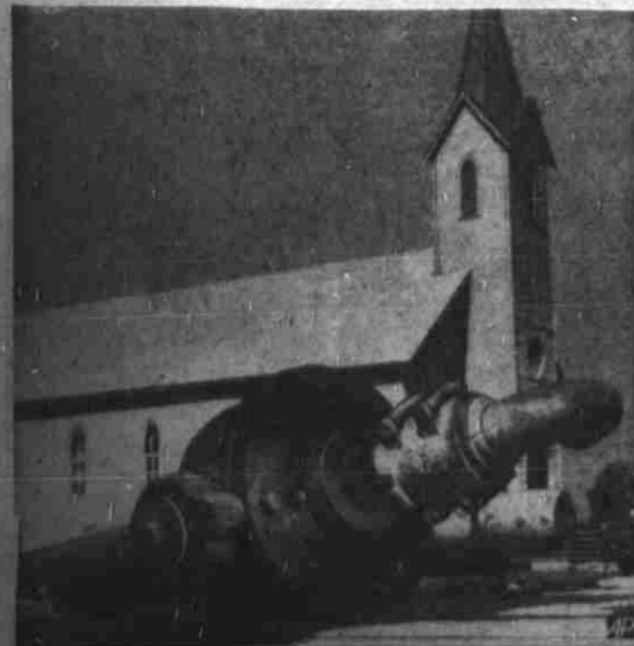
HELPS COLLECTIONS —Even the churches share in the boom oil has brought St. Elmo and other southern Illinois towns. One church reports $12,500 in royalties. Above, at St. Elmo, a giant swivel awaits drilling operations.
