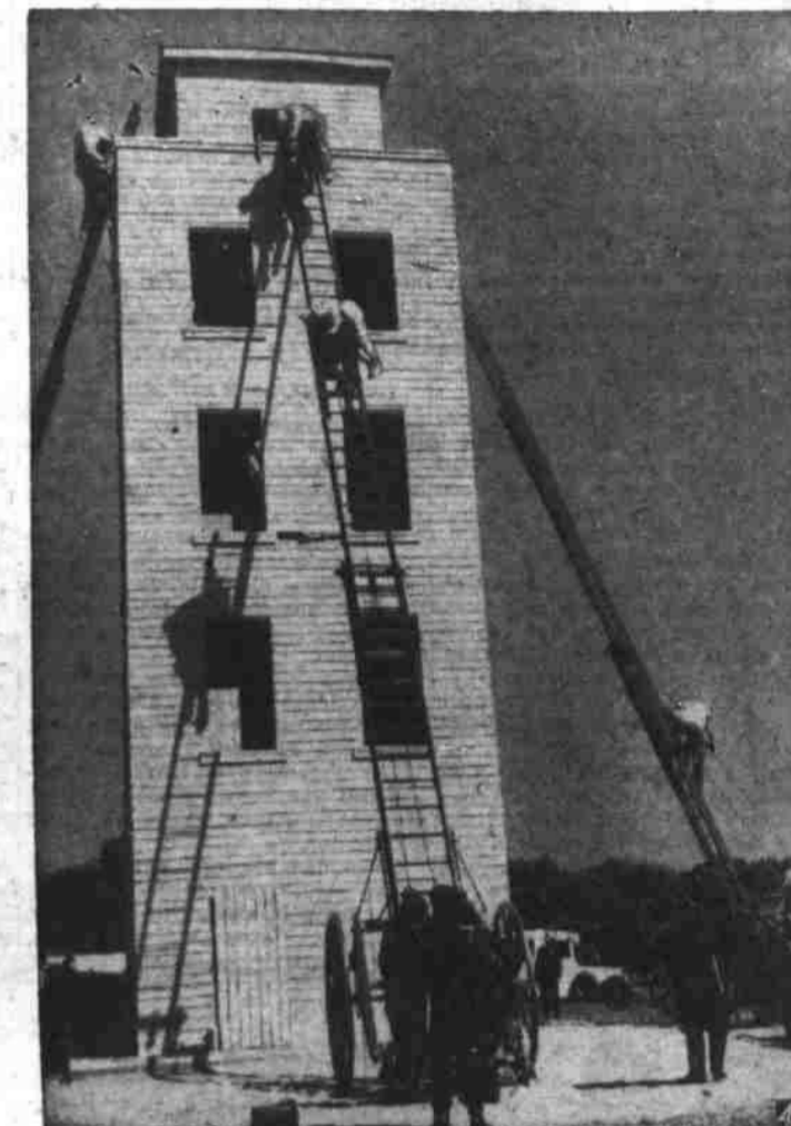
ONLY A REHEARSAL —Down the ladders climb members of London's fire brigade, as these firefighters show the Duke of Kent how they'd perform "under fire." An oil fire was extinguished with air-foam, during the demonstration.
