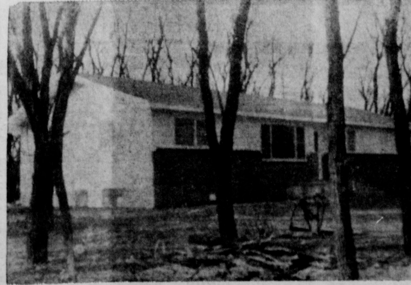
NEW HOME of Mr. and Mrs. Alva M. J. Davis recently completed under the Farmers Home Administration program.
