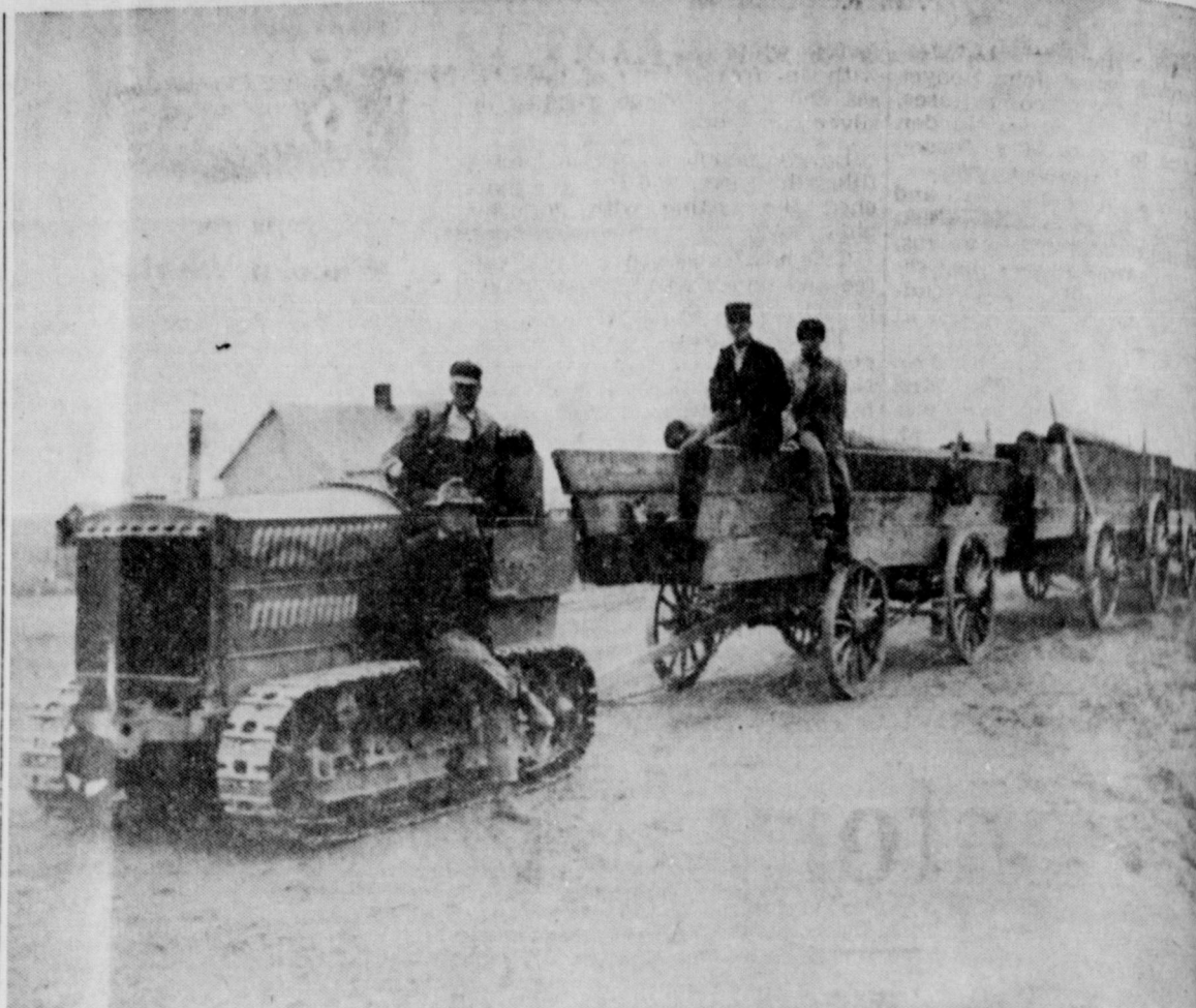
WAGON TRAIN—BUT NOT TV STYLE: These three wagon loads of lumber were hauled from Texola, Okla., as there was no bridge lumber available here, to build the bridge on Sweetwater Creek East of Wheeler in 1923. Pictured right to left: Jim Richards, W. O. Miller, Bonner Smith (on cat) and Pat Patterson (deceased). W. O. Miller was County Commissioner at that time.
