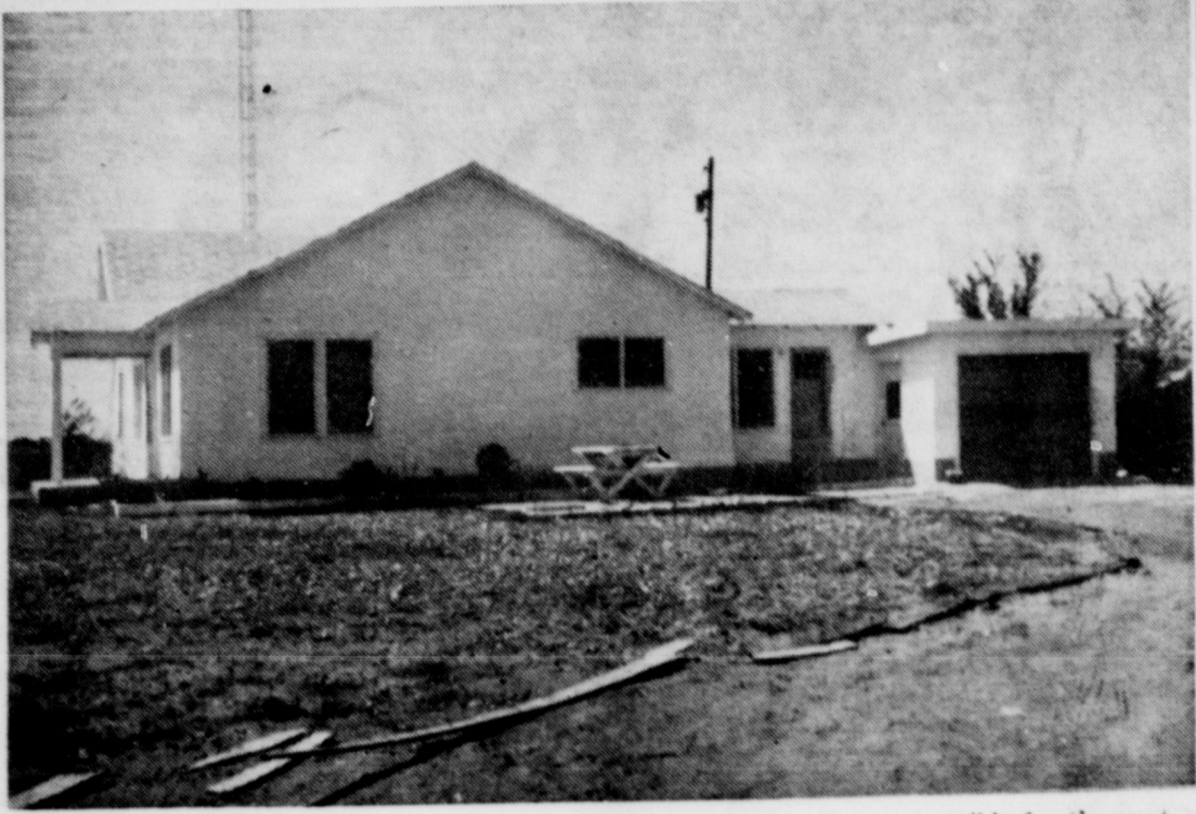
NICE IMPROVEMENTS: Carroll Adams and J. D. Wallace are responsible for the neat appearance of this house owned by Ed Riley and located about 1/4 of a mile West of Wheeler on the Farm to Market road. Adams and Wallace just recently remodeled the home for Riley.
