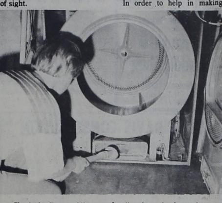
Check the Dryer while open for lint-clogged exhoust ducts.
