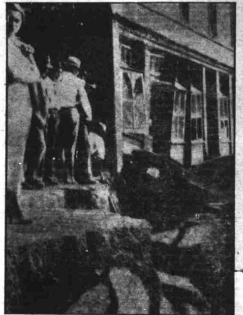
Undermined by recent floods of the Ohio river, a 225-foot stretch of Front street at Smithland, Ky., along the river bank was sinking gradually into the stream. River front buildings were damaged as shown above. Engineers planned to drive piles in a move to halt the cave-in. (Associated Press Photo)
