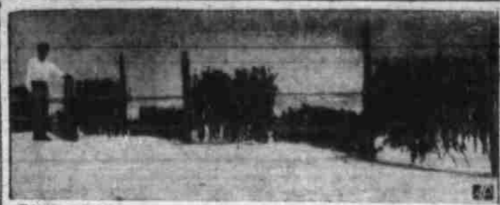
SAND TRAPS These checkerboard fences are being built along North Carolina's outer banks to anchor the sand and build a new shoreline for the government's proposed coastal park.
