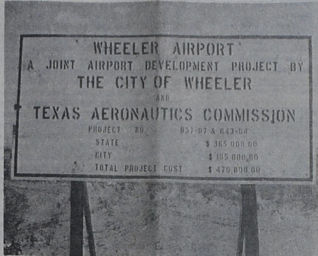
SIGN: This sign is located at the site of the new Wheeler Airport. Work is underway to lay the paving for the 3400 foot landing strip.
