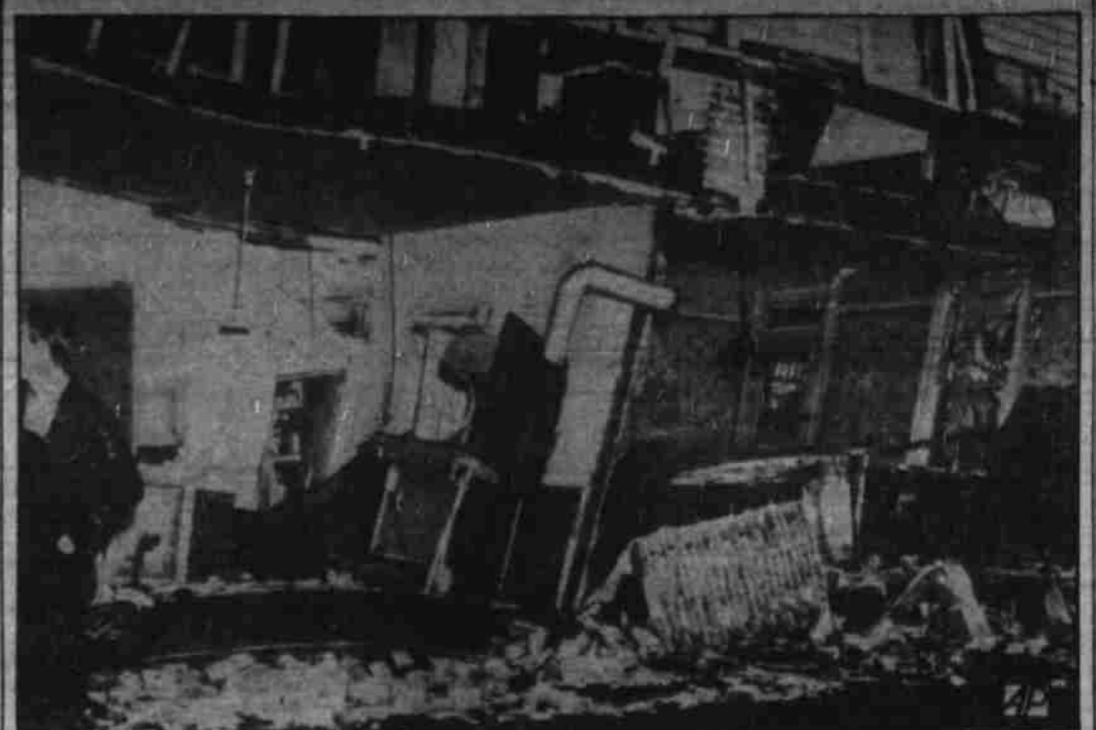
This Belleville, Ill., home virtually was demolished by a tornado which leveled houses in the city and left at least eight dead. The wall was ripped off this house and the interior wrecked.
