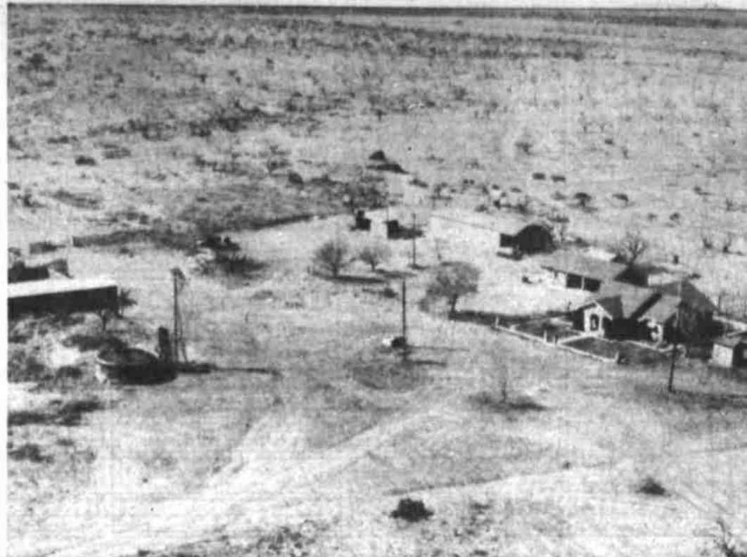
'SHOWPLACE' NEAR VINCENT Big rock home constructed in 1948
