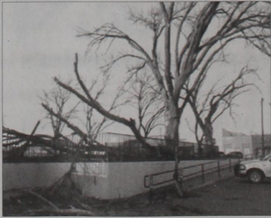
FRIDAY'S WIND DAMAGE: A large limb from a tree on the north side of the courthouse square was broken off by the front that moved through Wheeler Friday. No cars were parked in the area when the limb fell.
